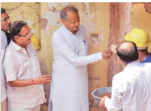
Rajasthan CM Ashok Gehlot launches renovation works at a stepwell under Indira Gandhi Shehri Rozgar Guarantee Yojana, in Jaipur on Friday PHOTO: PTI
